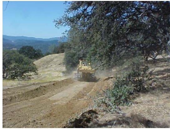
Bulldozer works on road extension (before and after)
