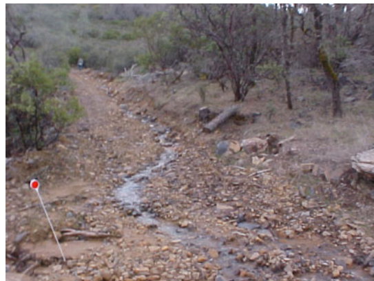
Drainage Improved and Road Widened Along the Entire Length
